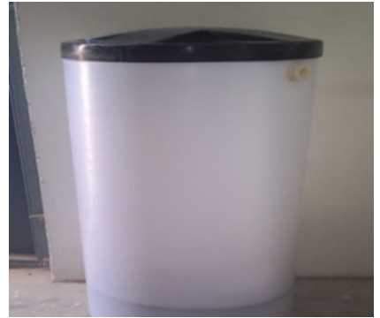
SALT TANK FOR REGENERATION It is the process through which the softener flushes out the minerals it catches from the hard water
